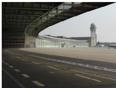
The monumental airport terminal of Tempelhof.
